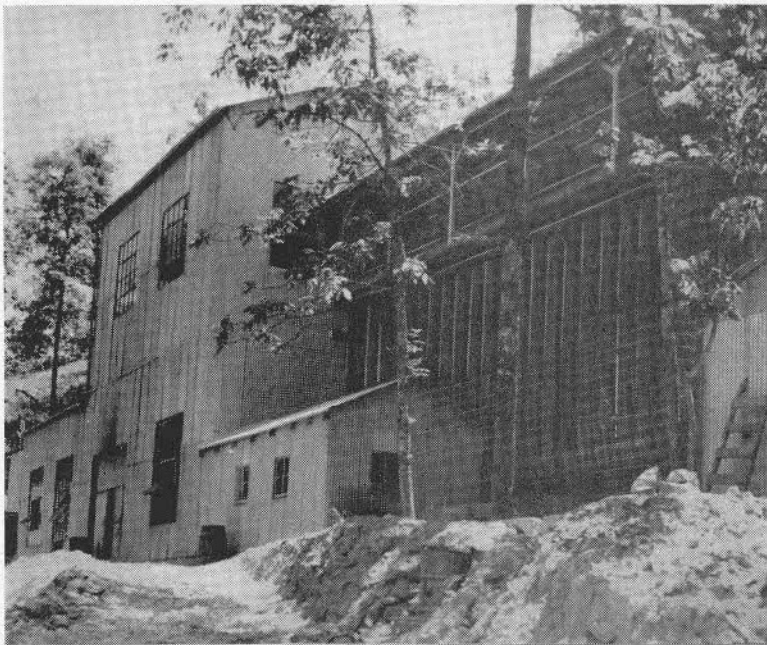
Furnace house and condensing system, Mercury Mines, Inc., Amity.
